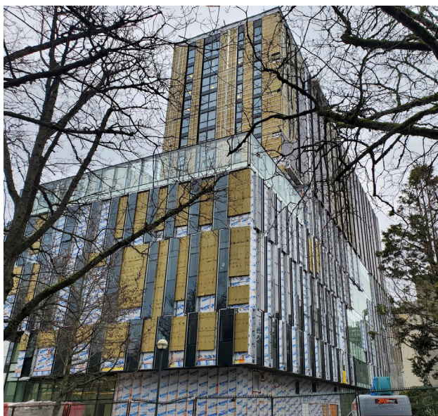
Above: Photo of Brock Commons in progress.
