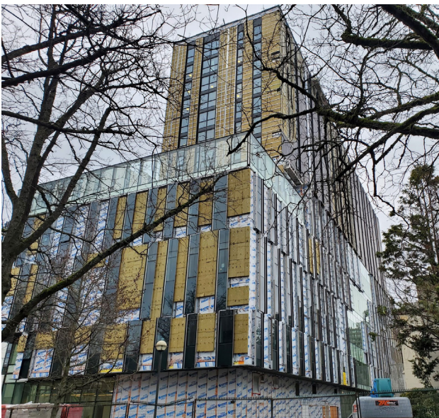
Above: Photo of Brock Commons in progress.
